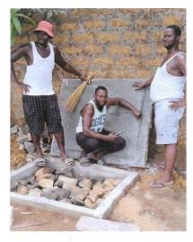
the angle of the pipe is right to send overflow into suck-away
